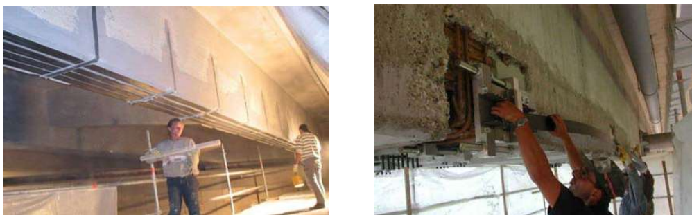
Figure 1. Two examples of the application of CFRP-strips to a bridge construction (HP-TL); left: Retrofitting by adhesively bonded slack CFRP-strips; right: Post-strengthening using a pre-stressing system.
