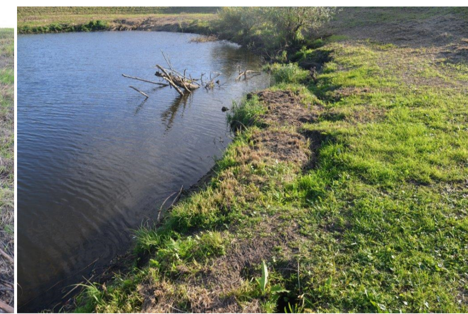
Figure 3 – Failure foreland sections due to beaver-caused cavities (Photo: Krüger)
