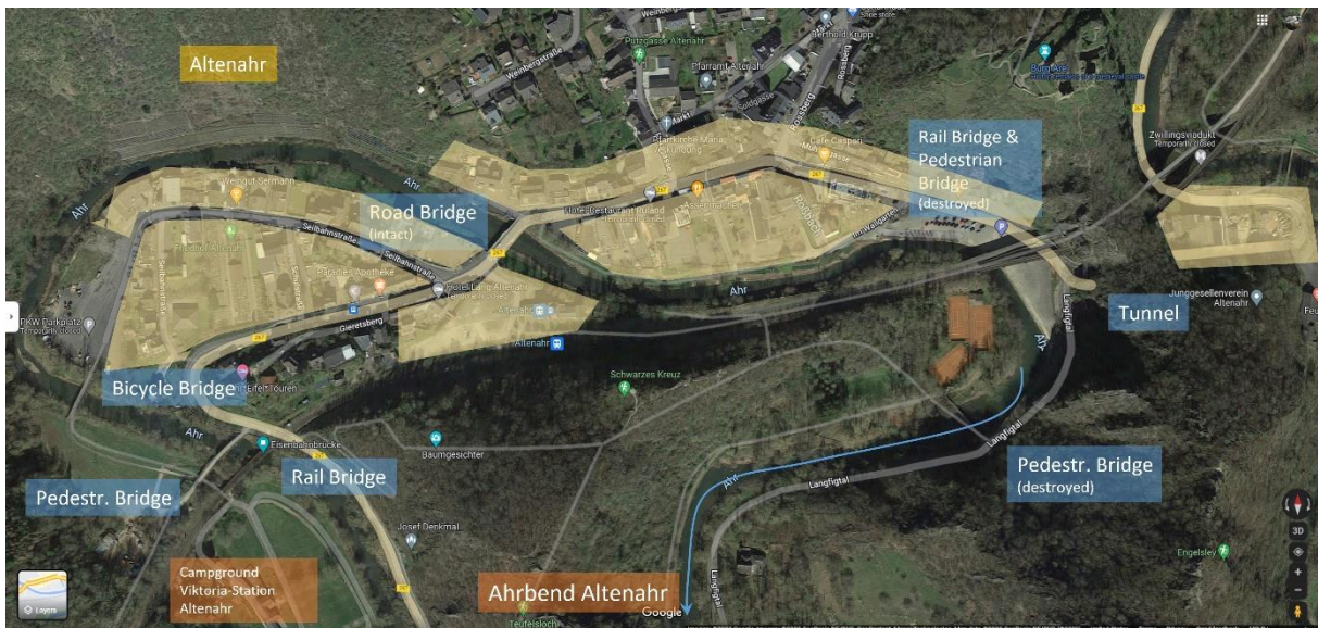
Figure 3. Aerial map of Altenahr with heavily flood damaged areas.
