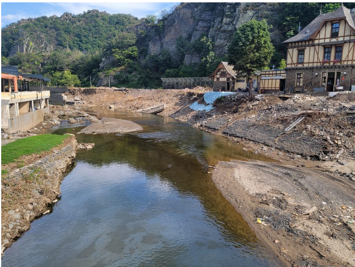
Figure 5. Soil erosion and retaining wall failure at the Altenahr train station.
