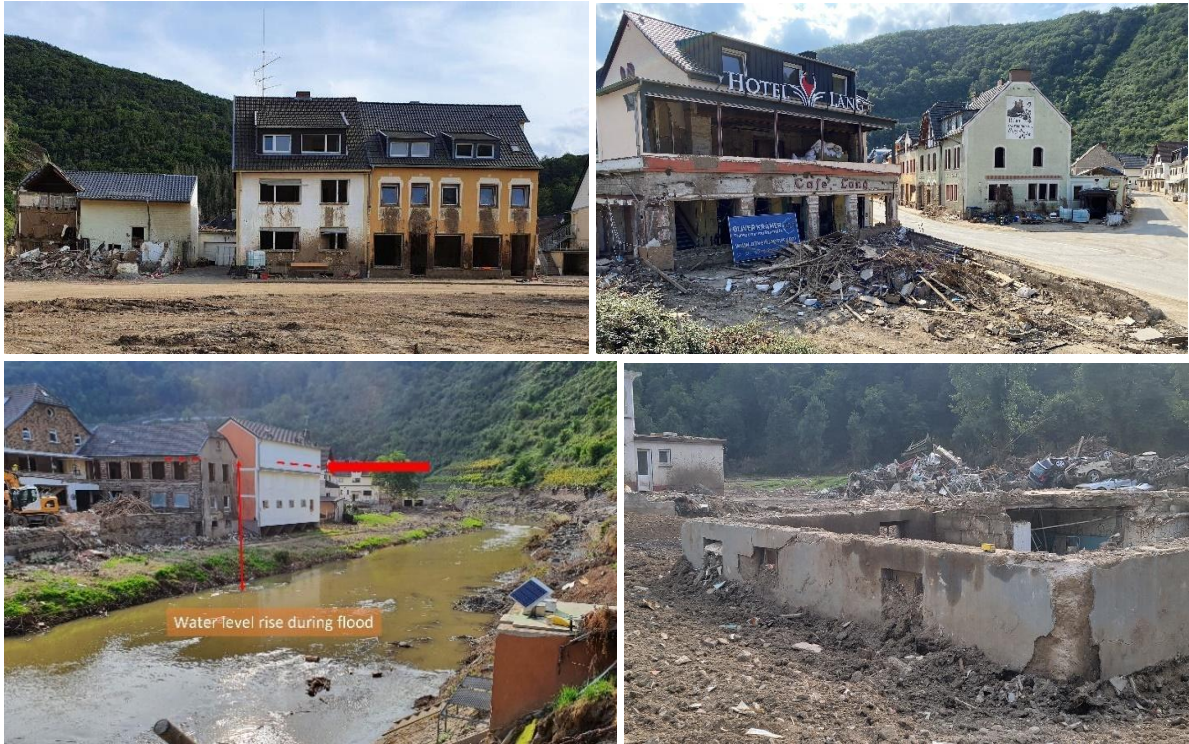
Figure 4. Example of structural/residential damage in Altenahr (town).
