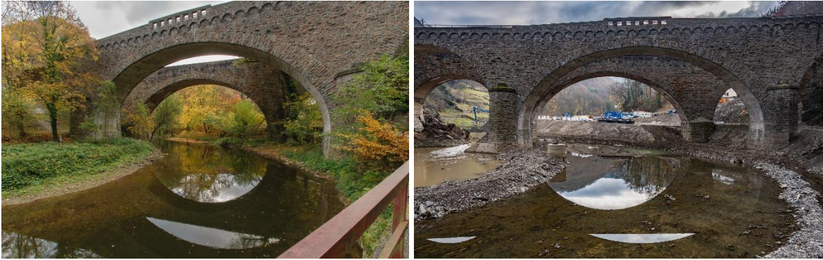
Figure 11. Before and photos of double bridge at tunnel exit taken in upstream direction, photo credit: Heinz Grates, Source and access at https://www.aw-wiki.de/w/index.php?curid=67031 ; Left: Pre-flood, Right: Post Flood and post-river rerouting back into its original riverbed
