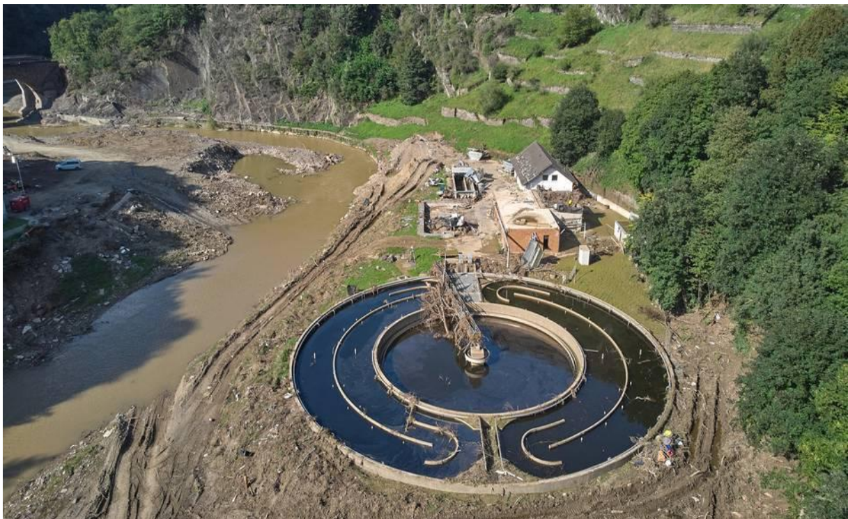
Figure 14. Wastewater treatment plant Altenahr following the 2021 flood, Source: DPA/Thomas Frey
