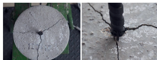
Figure 7: Splitting failure at UHPC | photos: Frank Schladitz
